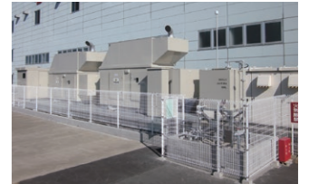
Emergency generator ensures a stable supply of electricity
